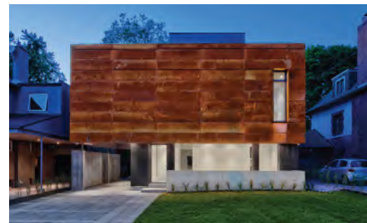
4.2.2(d) Consider how metals, weathered steel and other industrial materials can be used to evoke rail heritage and celebrate the Railway Transition Zone as an historically industrial district. (Fig. 81: Design Milk 2020)
