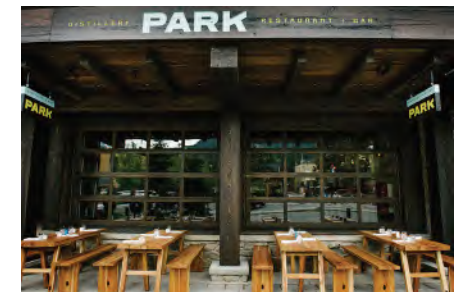
4.1.3(f) Consider the use of permeable garage-style doors, which can be opened in warm weather to allow interior activity to spill into the public realm. (Fig. 39: Park Distillery)
