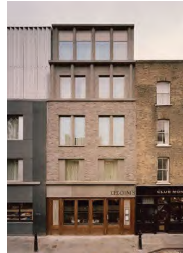
4.1.1(a) Upper-storey stepbacks used to accommodate additional height while fitting in with the older building next door (Fig. 30: 3144 Architects, 2019)
