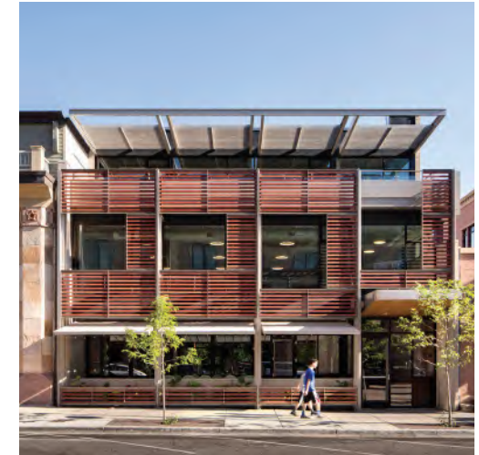
4.1.1(a) Vertical columns and pedestrian-scale overhangs to convey small storefronts at ground level, and an upper-storey stepback used to accommodate additional height (Fig. 31: Arch11 2020)
