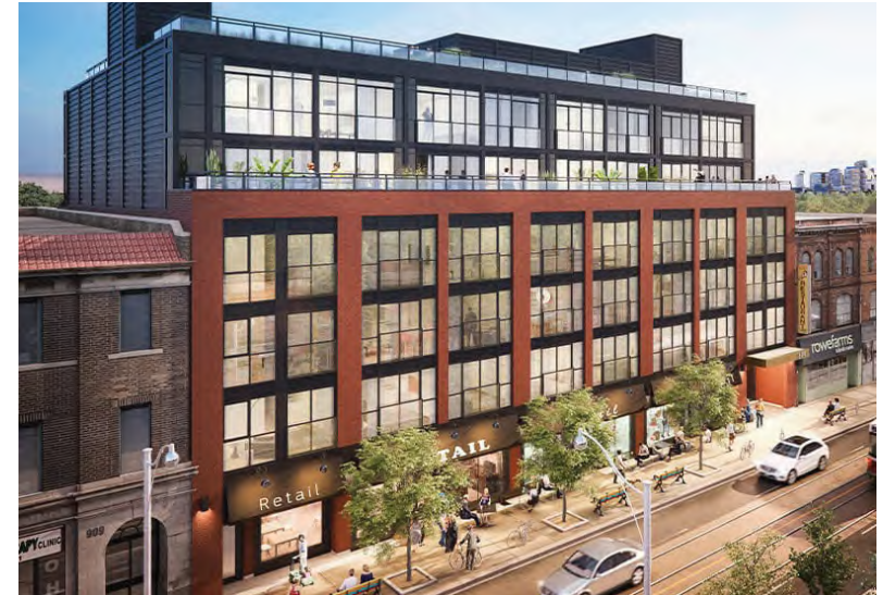
4.2.3(a-b) Site buildings with little-to-no setback from the front property line, and use strategies like upper-storey stepbacks to minimize heights greater than 4 storeys. (Fig. 85: Daniels Gateway Rental Communities)
