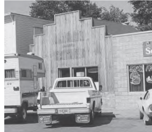
4.1.4(d) A false-front parapet was an historic method of converting a residential building (with a pitched roof) into a commercial storefront. The false front was meant to make the building appear as though it had a flat roof. (Fig. 44: Glenbow Archives, PA-1599-573-107)
