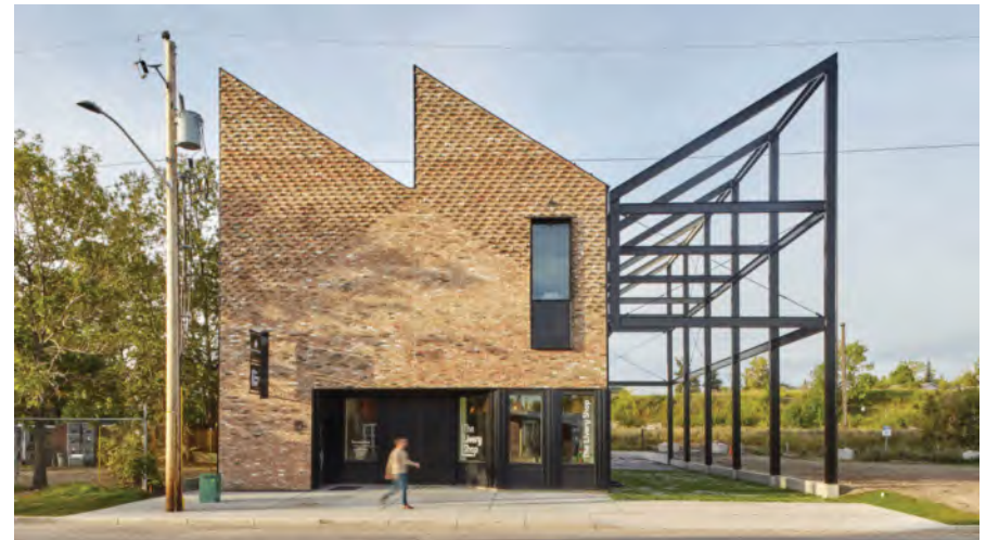
4.2.2(c) Buildings (and site landscapes) can be designed to create subtle interpretations of historic forms and themes, e.g. an interpretation of industrial railway-side building forms. (Fig. 80: Robert Lemermeyer, 2019)
