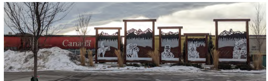
4.2.1(b) Upgrade barriers with creative aesthetic treatments to frame, highlight and celebrate rail corridor views. (Fig. 77: ERA 2020)
